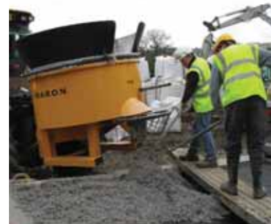
Limecrete slab being laid at Grand Designs' Carmarthen House.
